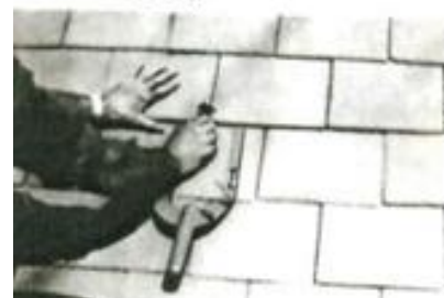
Two slate removed to show Snow-Guard fastened in place. However, slate does not have to be removed to install Guards.
